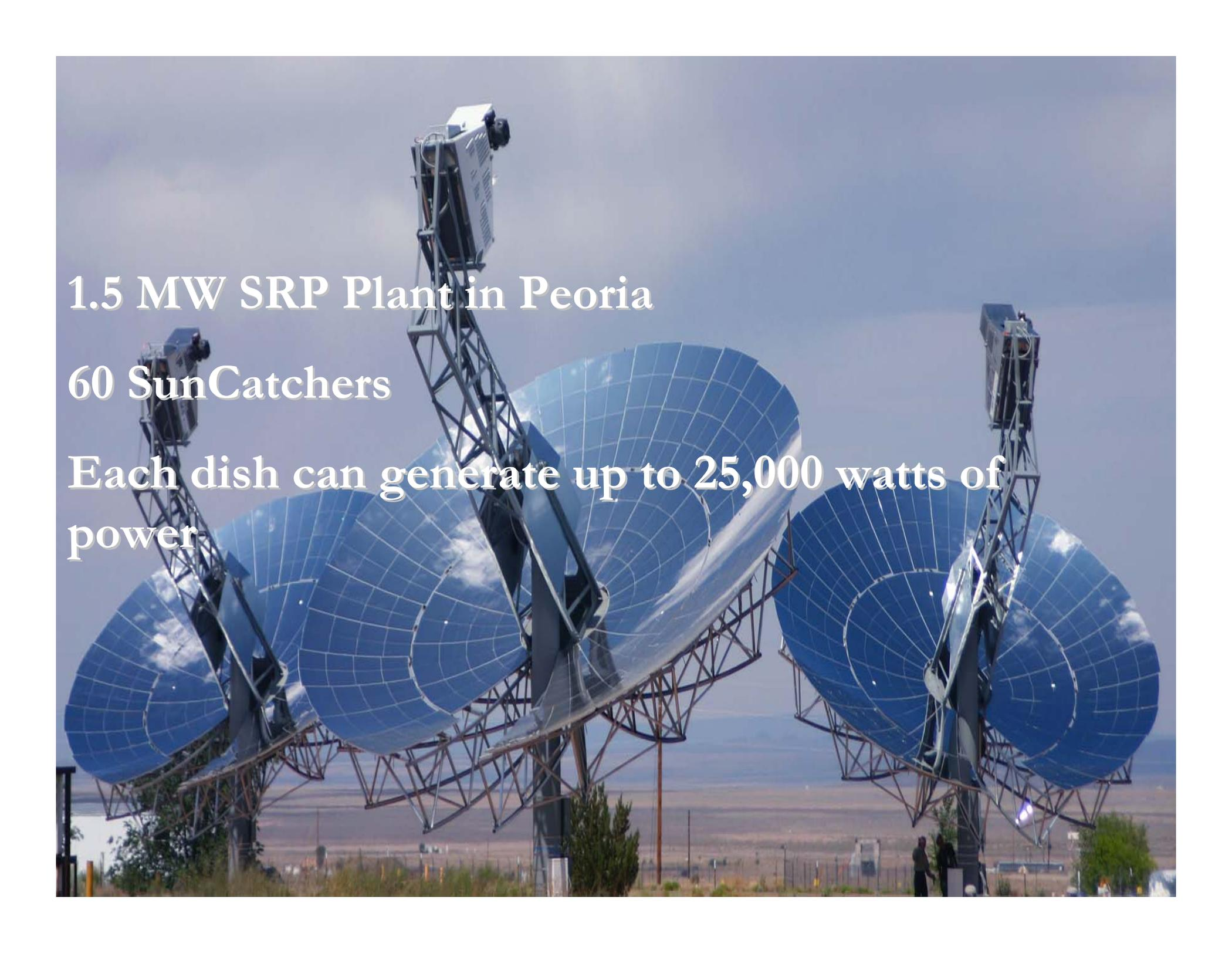
The image shows three large, blue, parabolic solar dish collectors (SunCatchers) mounted on metal structures. Each dish is supported by a complex metal frame and has a receiver at its focal point. The dishes are set against a clear blue sky with some light clouds. In the background, a flat landscape with some vegetation and a fence is visible. The text is overlaid on the left side of the image.
